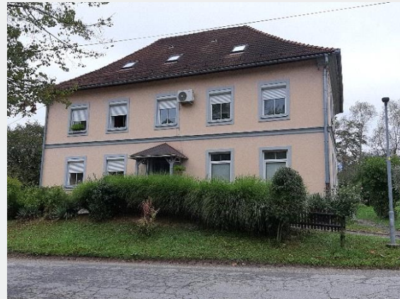
Primary school Vuhred (now a house of flats)
